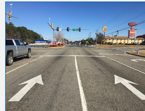
Northbound Approach (Route 15)
