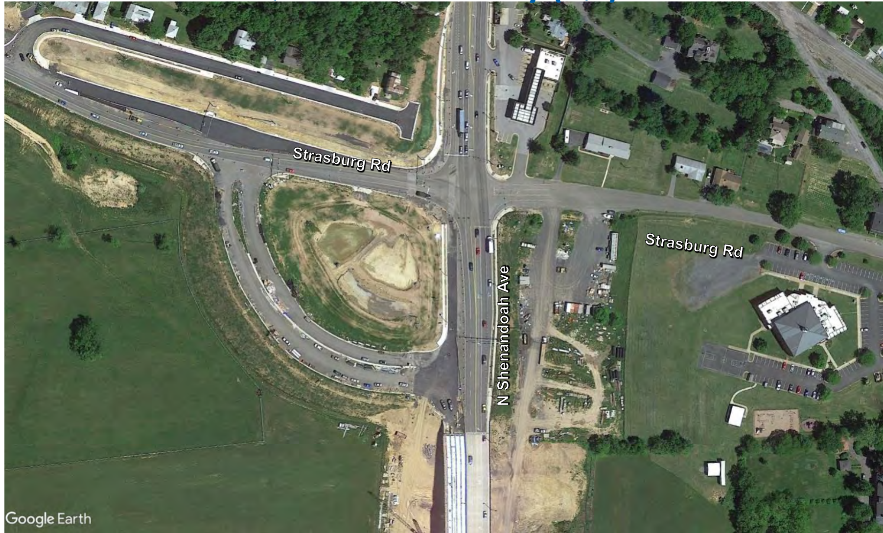
Strasburg Rd and N Shenandoah Ave, Warren County, VA – Under Construction
