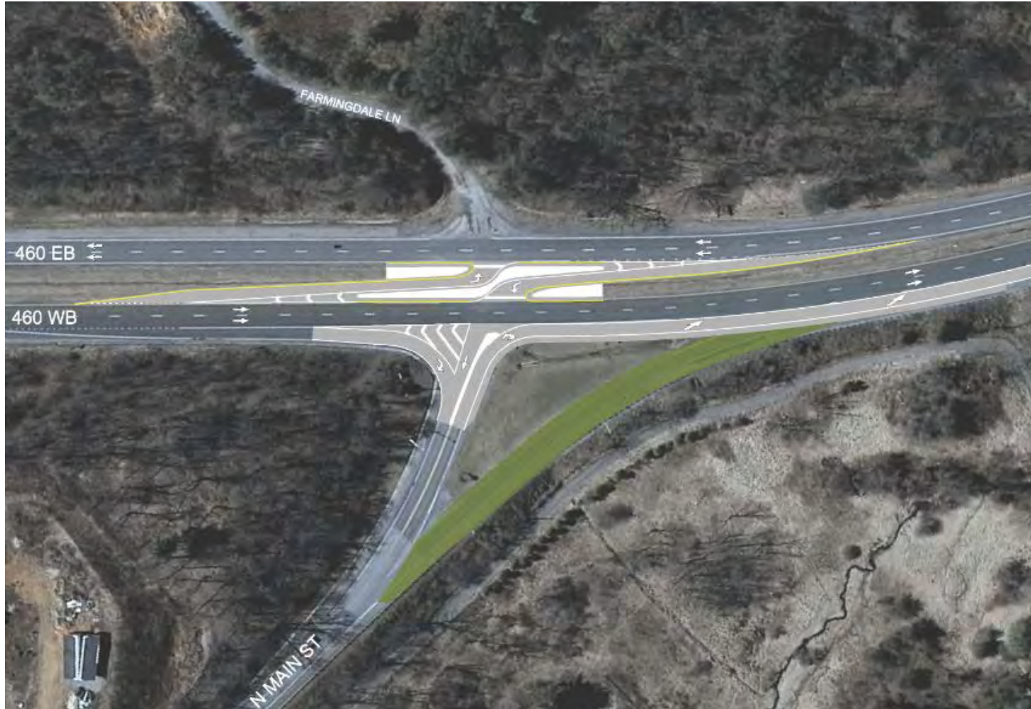
North Main St and Route 460 – Blacksburg, VA Est. Completion Fall 2018
