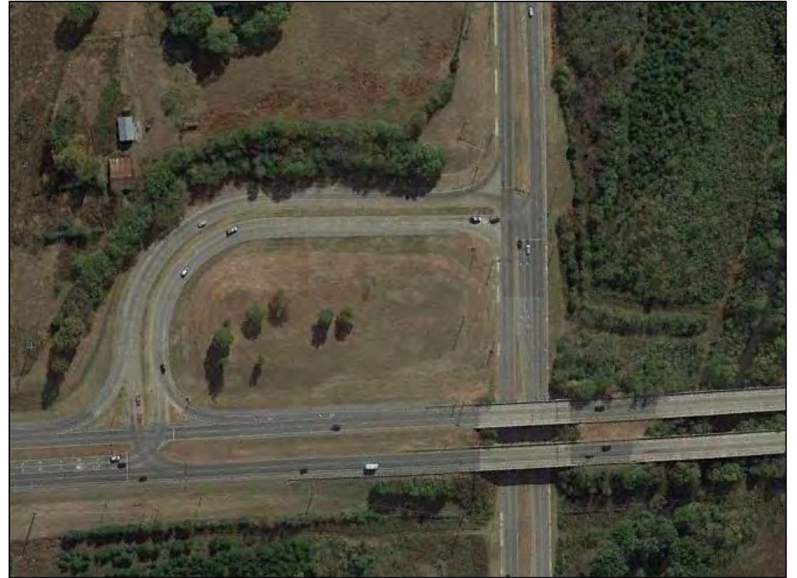
Grade Separated Quadrant at Lee Victory Pkwy and Old Nashville Hwy Smyrna, TN
