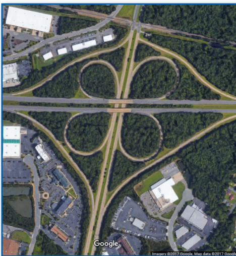
Interstate 64 over Airport Drive (Rt. 156)
