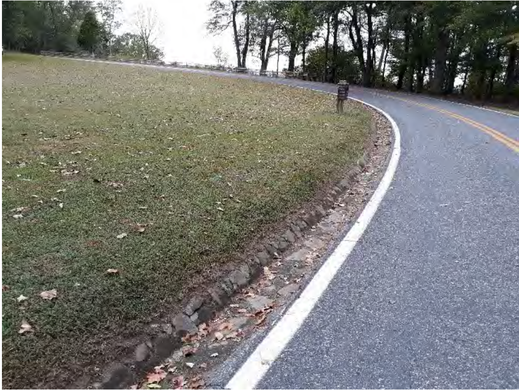
Figure 4. WPA Stone Guttering, Westmoreland County
