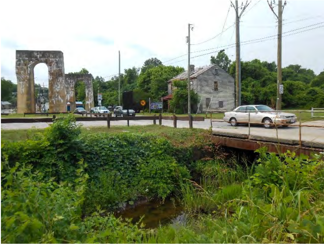
Figure 6. Bridge over an Historic Mill Race in the City of Petersburg
