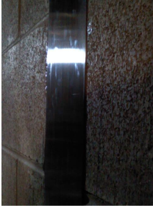
Figure 11 CFRP Plate bonded to a masonry wall
