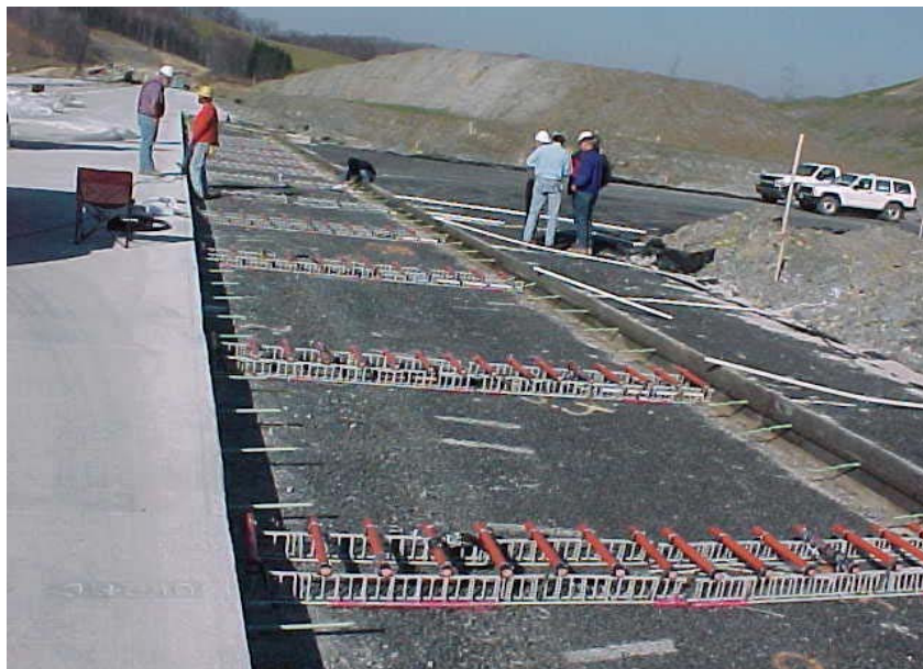
FRP dowels used for load transfer in concrete pavement
