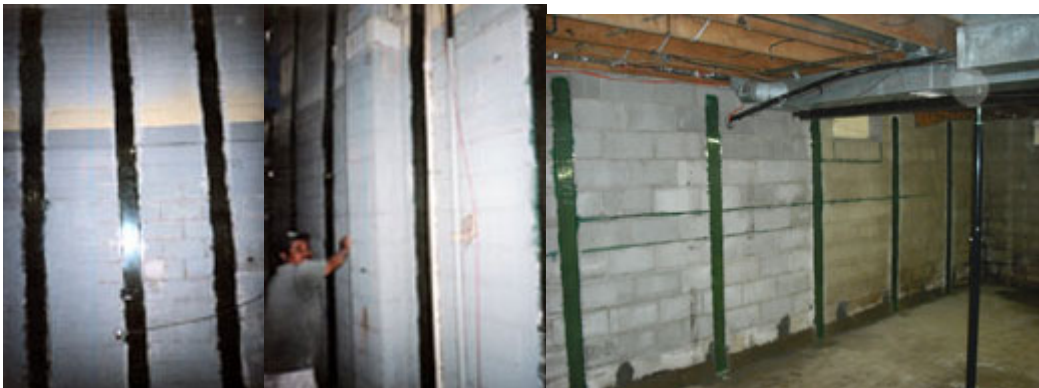
Images of carbon FRP plate (left) and carbon FRP grid (right) adhered to masonry walls for strength increase to resist bending loads
