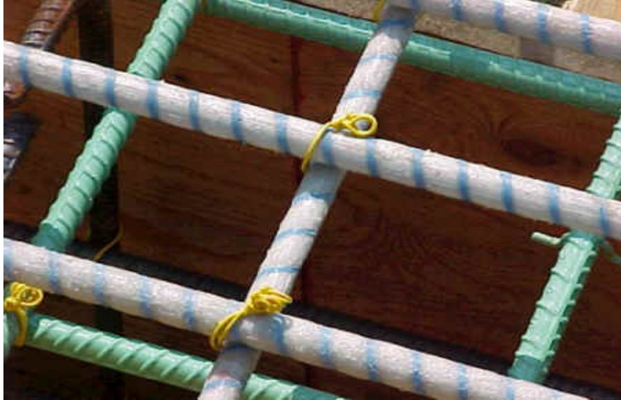
Glass FRP bars (striped bars) with epoxy coated steel rebar underneath
