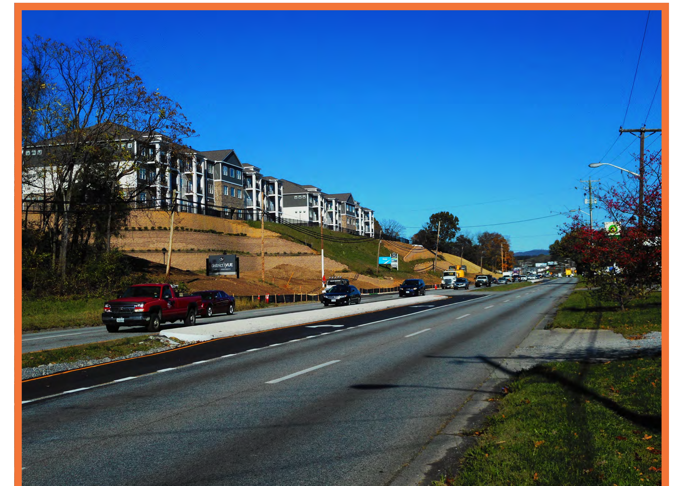
Median Crossover east of 24th St
